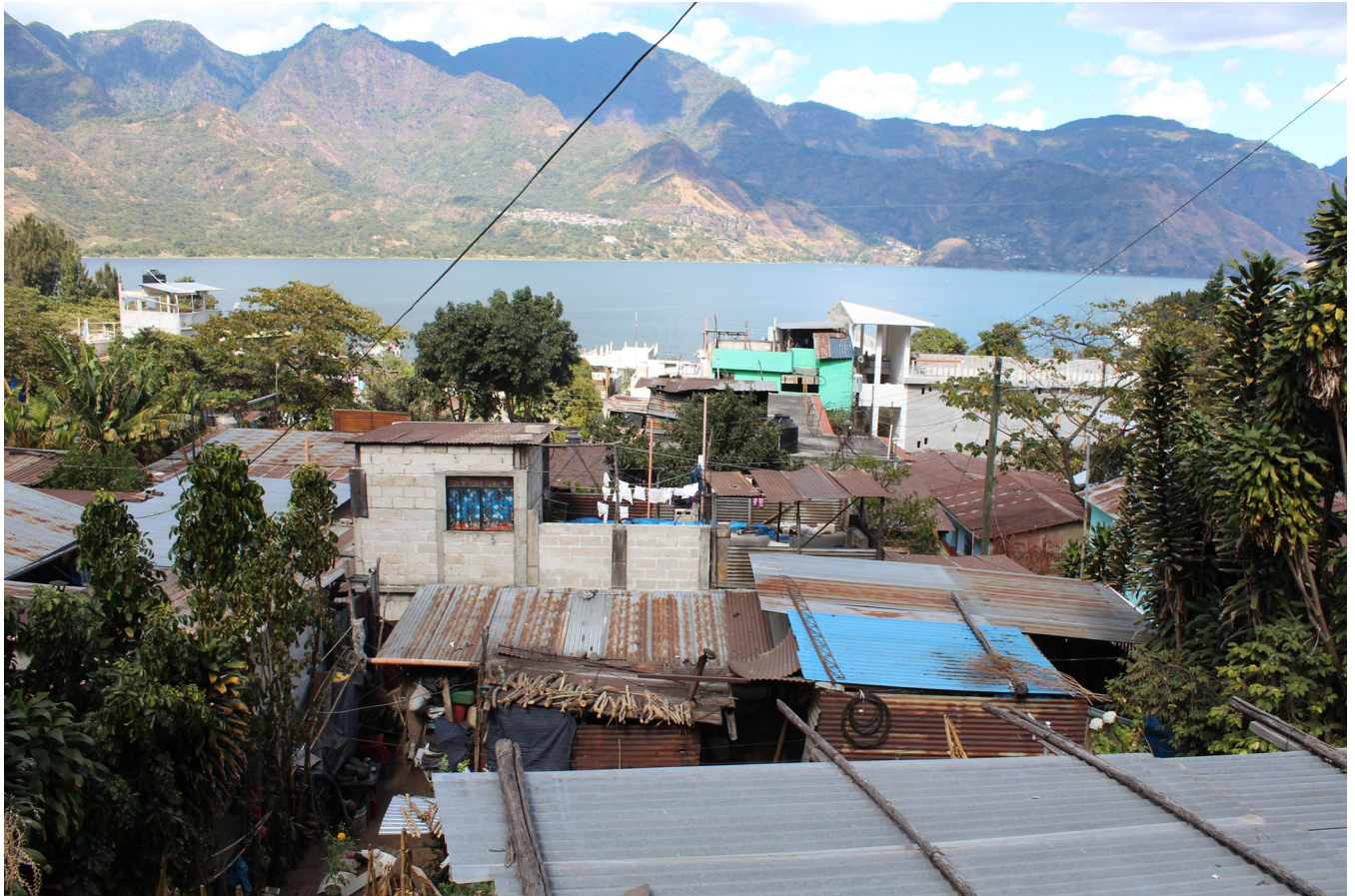
Fig 1. Houses in the Kaqchikel Maya community. The tin roofs that cover most houses are visible, and both adobe and concrete building material can be seen.
