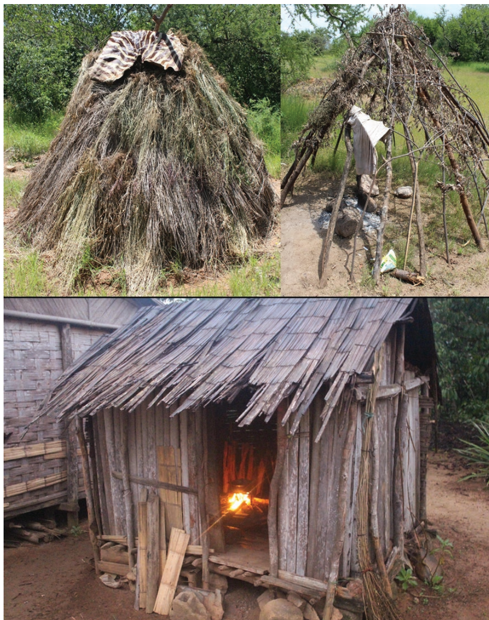
Figure 4. Top: Hadza home constructed from branches stuck into the ground (right) and then stuffed with grasses (left). Bottom: Malagasy home constructed from wood. Participant consent for photographs was given to DRS.
